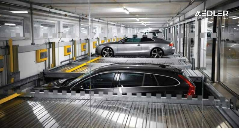
Semi-Automated systems make use of mechanical lift technology with the addition of electricals and PLCs to make the car platform move. The system works to store cars from 2 levels high up to a maximum of 6 levels. All parking places can be selected and used independently. The column-free construction ensures that vertical supports are only required at every 2 or 3 parking spaces next to each other.
